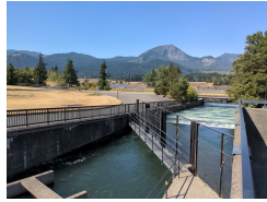
Fish ladder at Bonneville Dam
